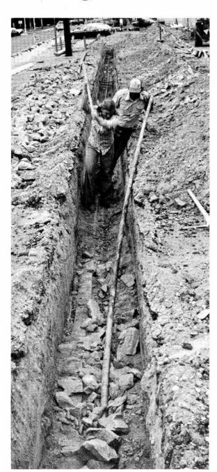
PICK & SHOVEL work is being done to remove and replace old, leaky steam lines. Plant Engineering estimates that more than a mile of such pipeline needs to be replaced.
